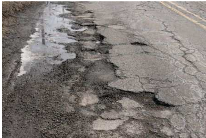
Example of road infrastructure condition
